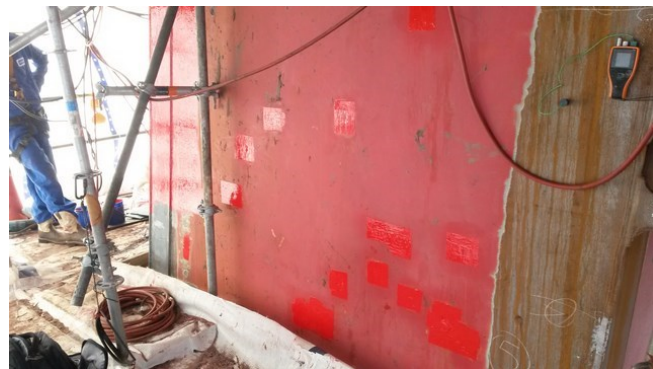
Humidur as coating repair system
