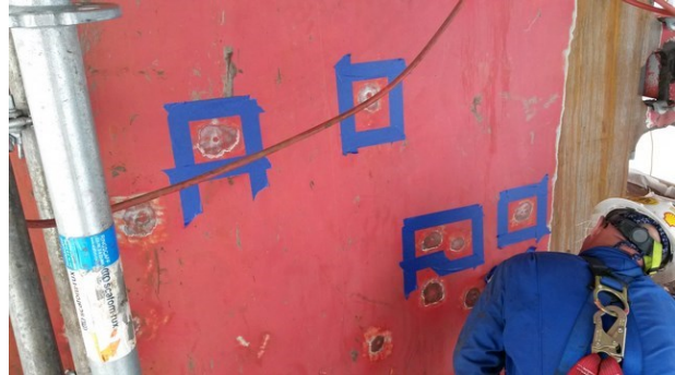
Repair of existing coating: St3 prepared surfaces
