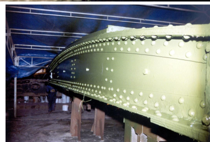
View on the sandblasted and coated lock door after dismantling
