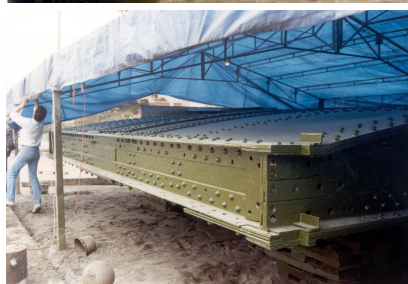
View on the sandblasted and coated lock door after dismantling
