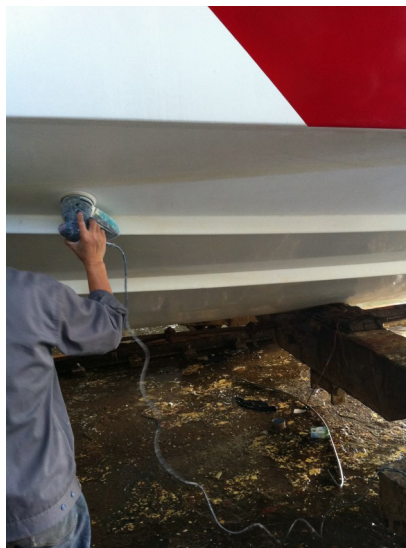
Surface preparation of GRP
