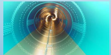
Interior hydropower pipeline
