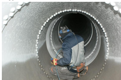
Final quality control on coated surface: visual, dry film thickness and spark testing
