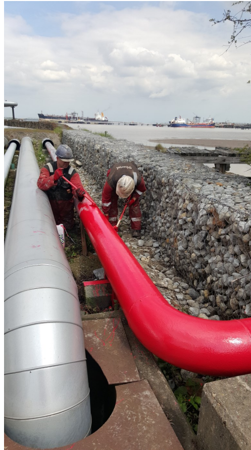
Fire water line coated with Humidur
