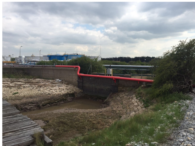
Fire water line coated with Humidur
