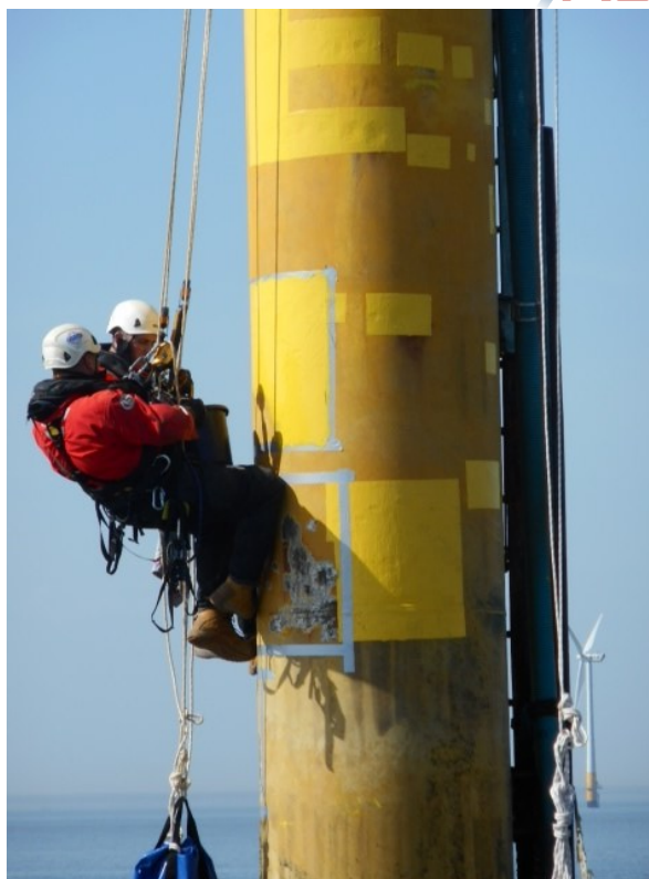
Coating repairs: rope-access
