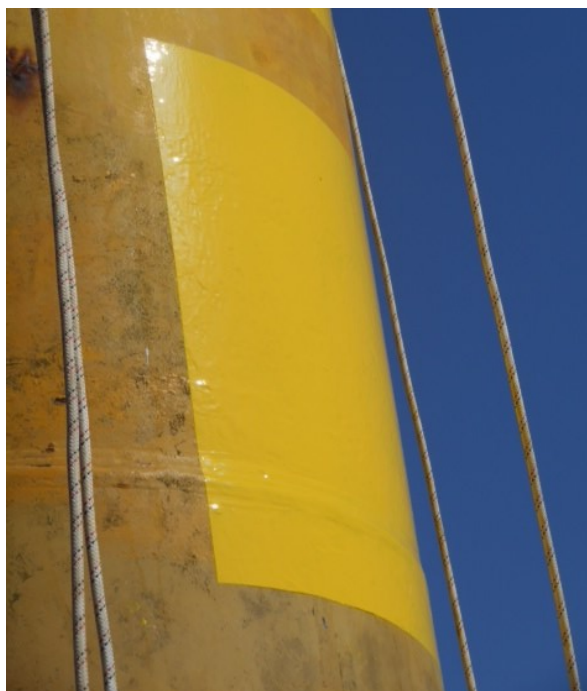
Coating repairs: rope-access
