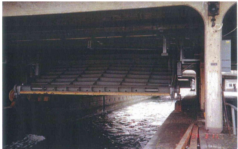
Different views on the coated and protected lock door in Stockholm
