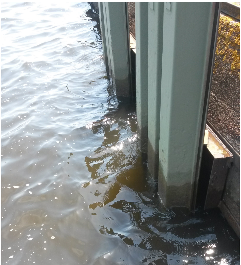
Coated sheet piles in excellent condition after 8 years of exposure to harsh environments (2015)
