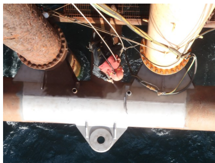
Abrasive blasting by rope-access
