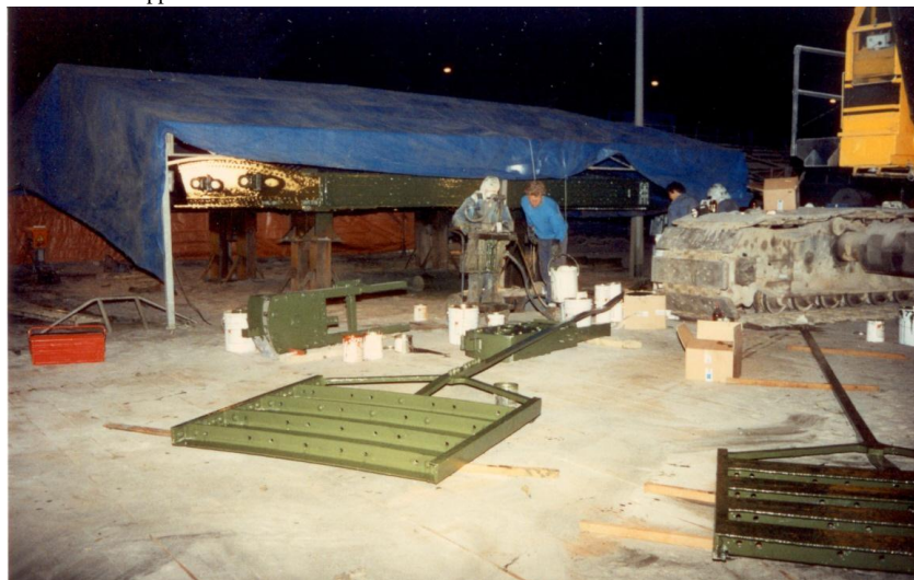
Smaller parts and covered lock door after coating application
