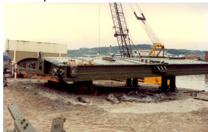
View on the sandblasted and coated lock door after dismantling
