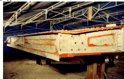
View on the sandblasted and coated lock door after dismantling
