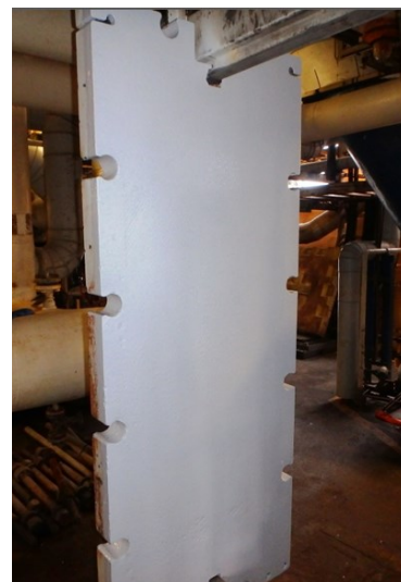
Coating repair with Humidur®
