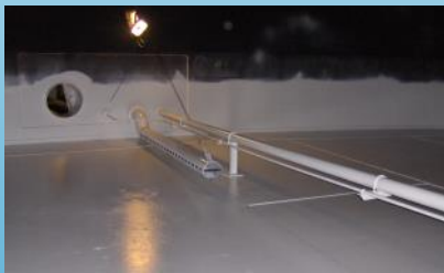
Interior crude oil storage tank
