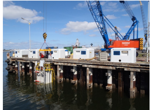
Treatment of tubular piles with cofferdam
