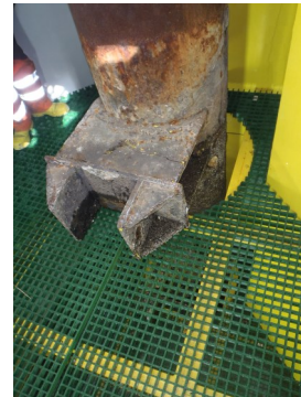
Inside cofferdam: before treatment, after cleaning and after coating
