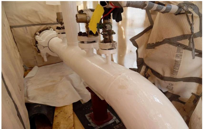
Pipeline coated with Humidur®
