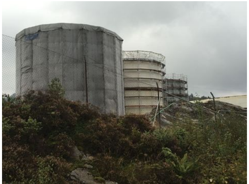
Tanks containing jet fuel A1 at Dolvik Depot, Bergen, Norway
