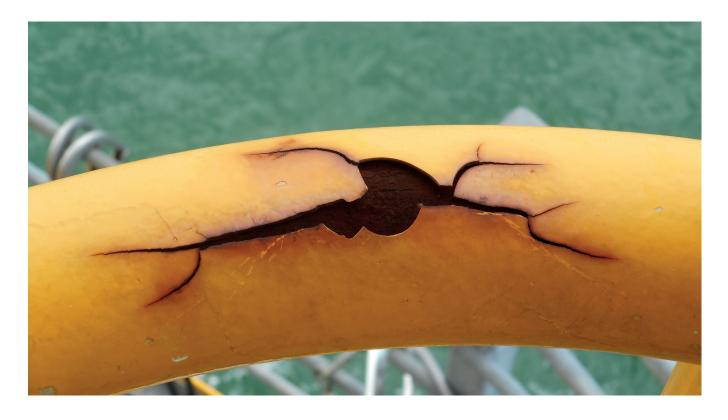
Offshore wind turbines suffer from severe corrosion and with limited access to them, the choice of the right corrosion protection is crucial. The most widely used protection methods are anti-corrosion coatings, often in combination with cathodic protection (in the submerged zone). However, these coatings often suffer from premature failure due to mechanical damage, application errors or the wrong choice of coating system.
