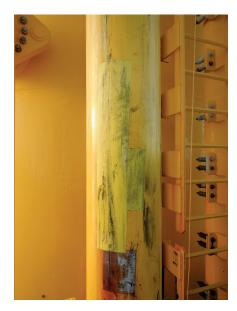
The coating is applied in one yellow layer, by brush at a thickness of 400 µm. The thickness during application is checked with WFT gauges. As the coating is a solvent-free system, the wet film thickness equals the dry film thickness.
