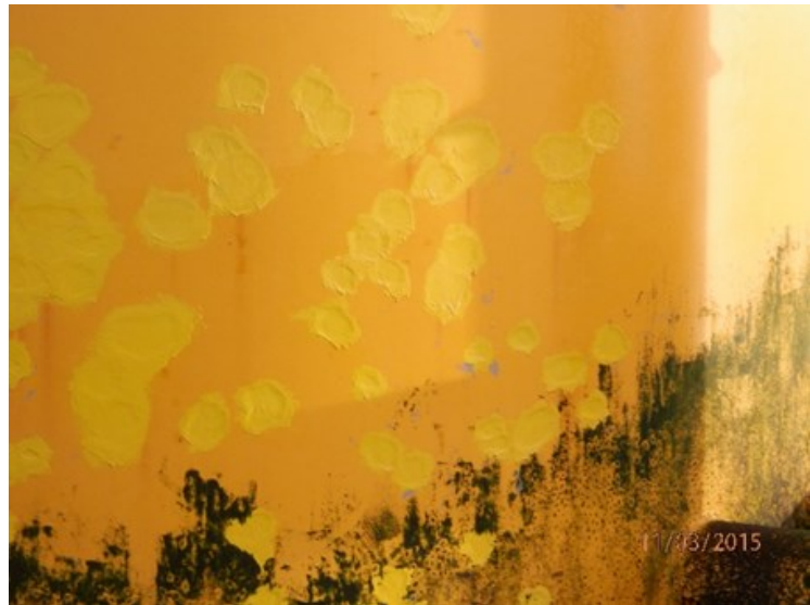
Repairs with Humidur®
