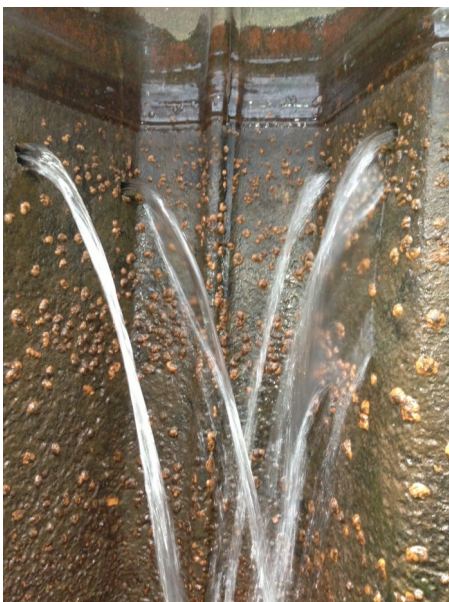
Severely corroded steel sheet pile
