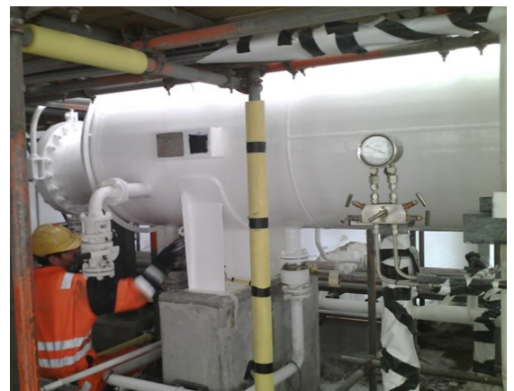
Methanol coalescer coated with Humidur® anti-corrosion coat and topcoat
