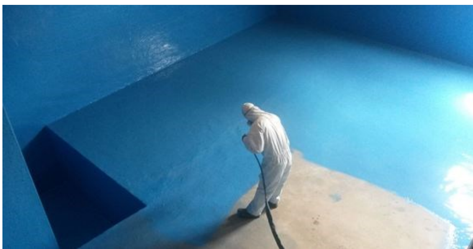
Application of Humidur® in a concrete tank for Backus SABMiller, Peru
