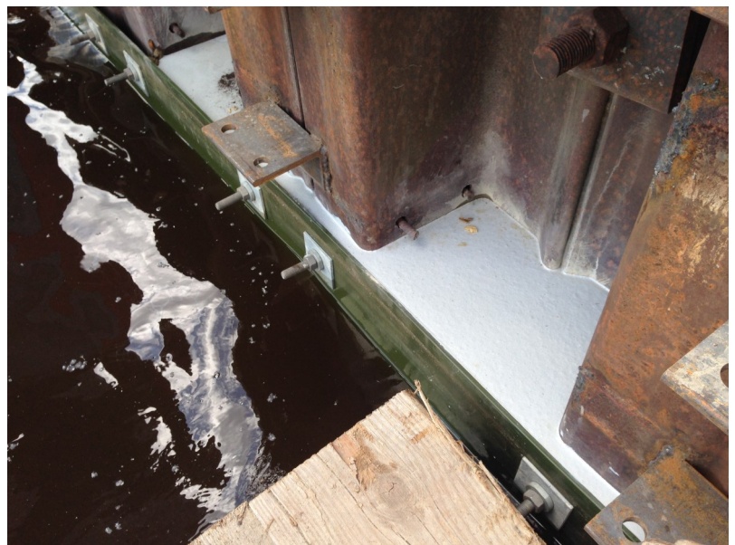
Rehabilitation sheet pile in Duluth, USA
