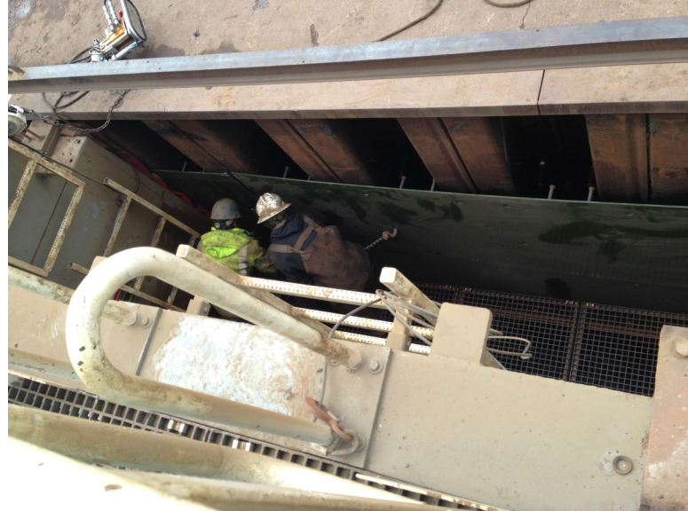
Installation of pre-coated steel plates by means of Acotec's DZI cofferdam
