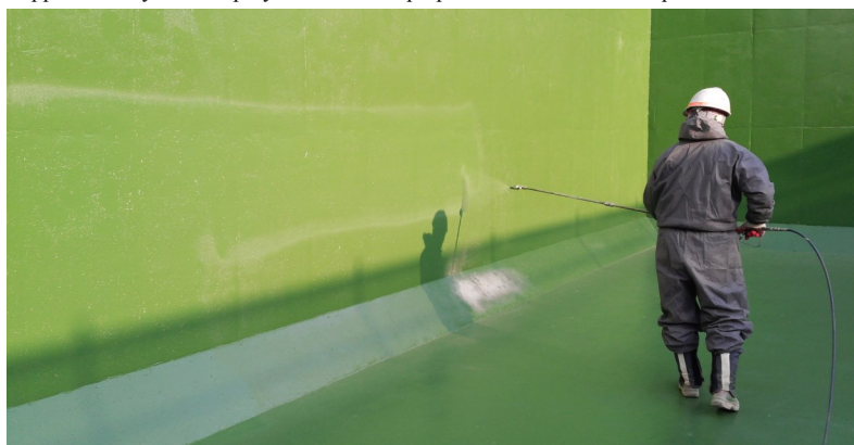
Application by airless spray after surface preparation of the concrete pond
