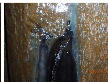
Perforation due to MIC in submerged zone
