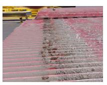
Fouling on the bar screen before surface preparation. Every year this was manually removed by divers.
