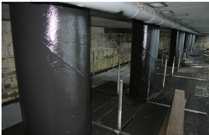
View of tubular piles after repair and anti-corrosion treatment with Humidur®
