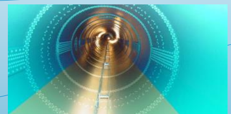
Interior hydropower pipeline
