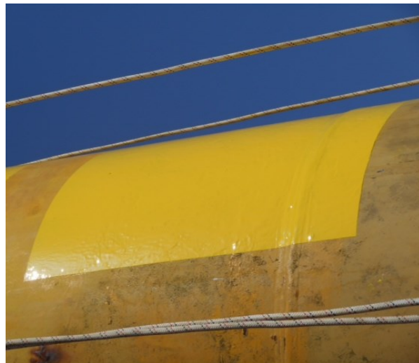
Coating repairs: rope-access
