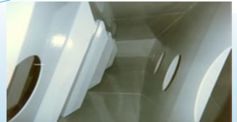
Ballast tank of an ocean carrier
