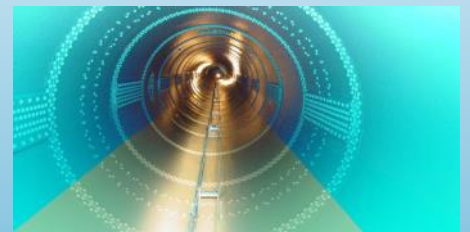
Interior hydropower pipeline
