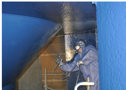
One layer of Humidur to protect the zone which will be submerged up to a DFT of 1200µm
