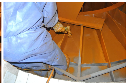
Coating work at locations which will be covered in oils and grease
