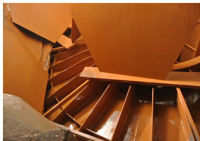
Coating work at locations which will be covered in oils and grease
