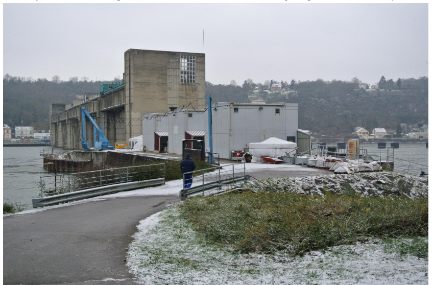
General overview of the Mericourt Kraftwerk
