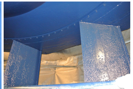
One layer of Humidur to protect the zone which will be submerged up to a DFT of 1200µm
