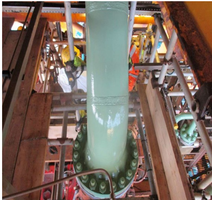
Coating repairs with Humidur®
