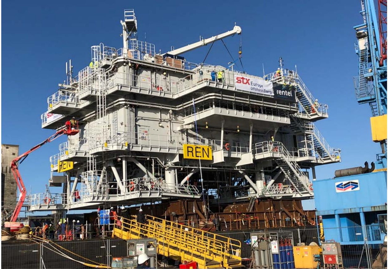
Photo 1: The offshore transformer substation in the assembly yard in Saint-Nazaire
